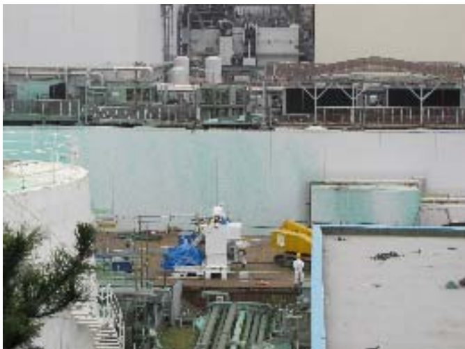
③ View from large crane around a reactor building Sep 15, 2011
