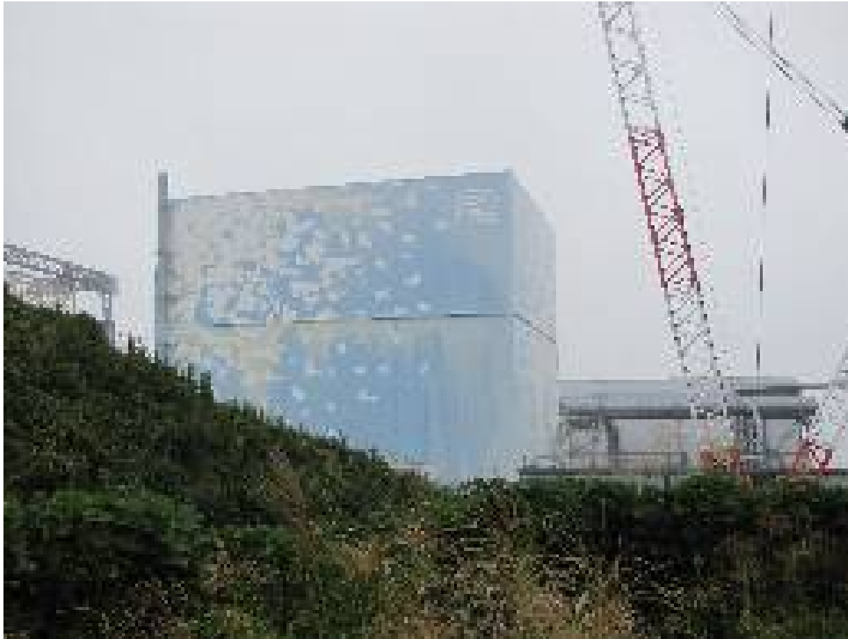
⑤ Overview of a reactor building from western hilltop Sep 15, 2011
