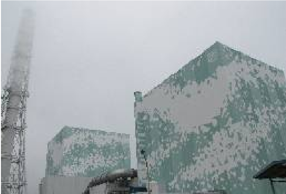
⑪ Overview of a reactor building from southwest side Sep 15, 2011
