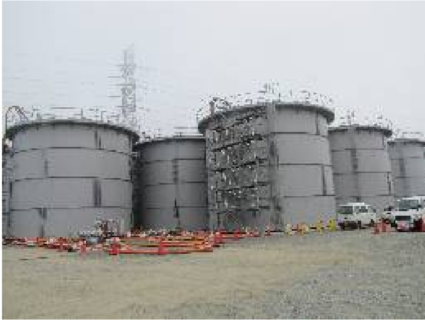
⑬ RO concentrated water storage tank (H1 east area) Sep 15, 2011
