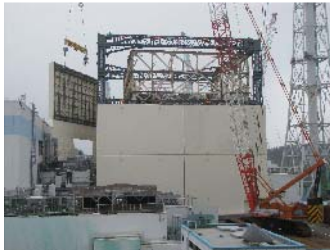
② Reactor building cover from northern side Sep 15, 2011
